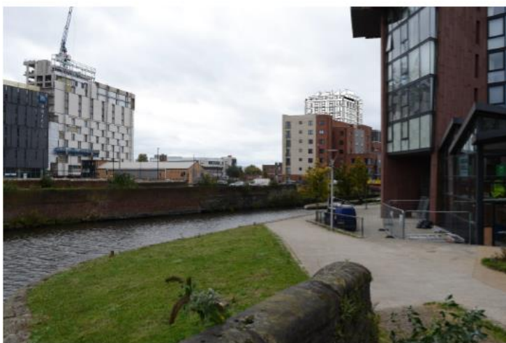
View 2 :The view south-westwards from the tow path bridge across the Islington Branch Canal
